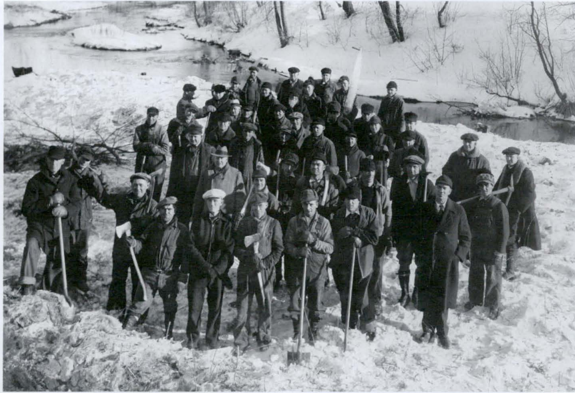
A Works Progress Administration work crew on a river cleanup project in Fargo, about 1936.
