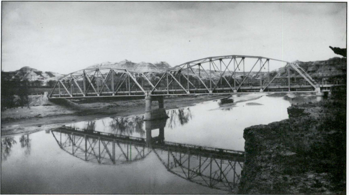
Two polygonal through-tresses provided an engaging bridge design set against the scenic backdrop of the Little Missouri River. No longer standing, portions of the bridge and its trusses were likely recycled in a later project elsewhere in the state.
