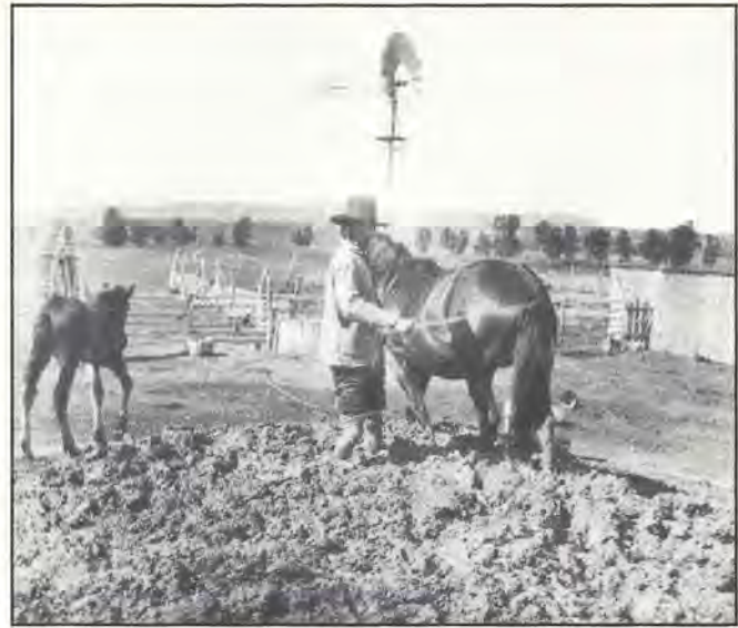
A man and his horse mixing mud to be used for plaster in western North Dakota, ca. 1900-1905.
