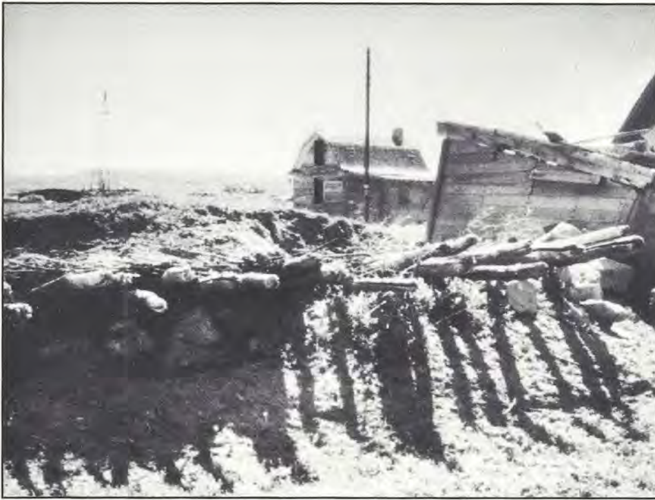
Based on the Russian prototype, a makeshift dwelling called a semeljanka was built partially underground, walled with clay, and featured an earth, wood or reed roof. The protruding logs formed the roof supports of this partially collapsed semeljanka at the Gross Farm in Emmons County. From the Division of Archeology and Historic Preservation files.
