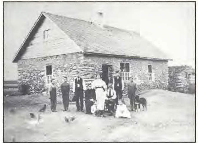
August Mantz home near Center in Oliver County. A settlement period scene shows a traditional house plan with a gabled roof and central chimney. This one is largely constructed of flat fieldstone.
