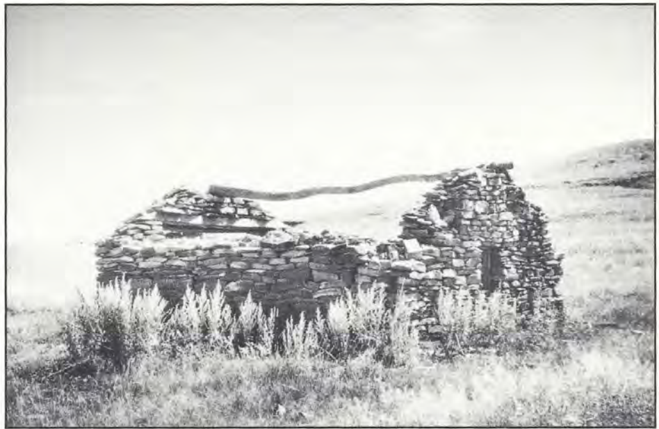
The roof support beam, or swolok, on this fieldstone structure has survived the decades at the Valentine Hutmacher farmstead in Dunn County. Courtesy of the author.
