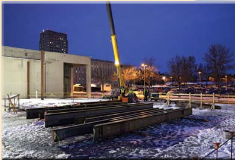
Work on the expansion of the North Dakota Heritage Center continues on schedule. (left) A construction crew stands ready in the early morning of December 7 to install horizontal steel beams, the framework for the Early Peoples Gallery , which will tell the story from the end of the last Ice Age about 12,000 years ago to the creation of Dakota Territory in 1861. Looming in the background is the 19-story state capitol tower. (right) As the morning sky brightens, the crew begins installing the horizontal beams.
