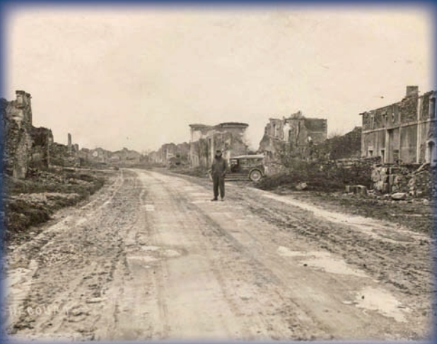
The badly damaged village of Richecourt in northeast France in 1918 or 1919.
