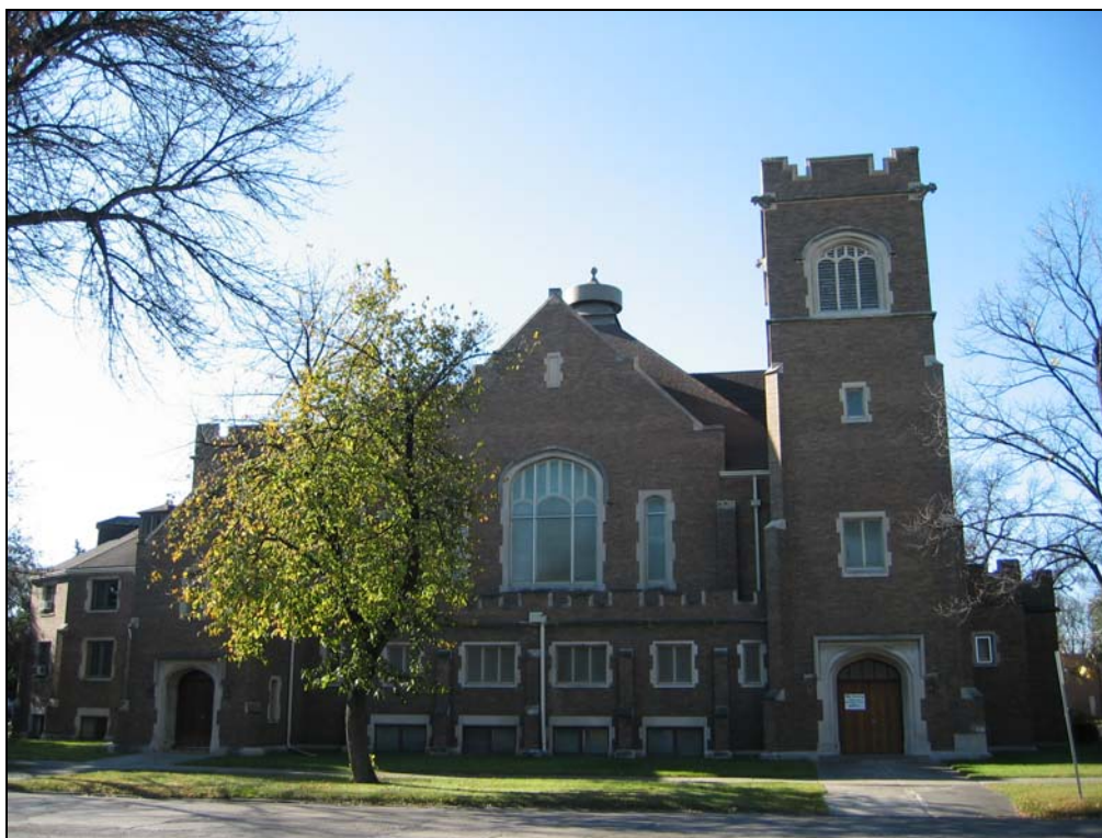
1 st Presbyterian Church (1910) in Grand Forks [photo taken by M.L. Dennis, 2011]
