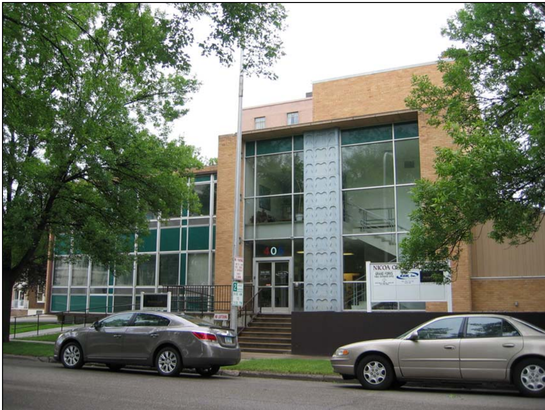
Implement Dealers Mutual Insurance Company Building (1954) in Grand Forks [photo taken by M.L. Dennis 2012]
