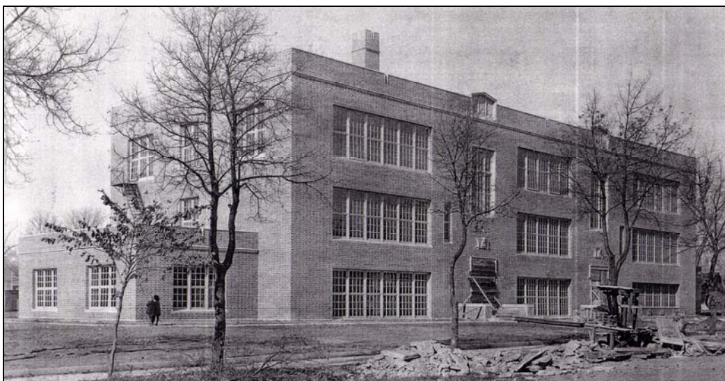
Photograph of Park River School near completion [photographer unknown]
