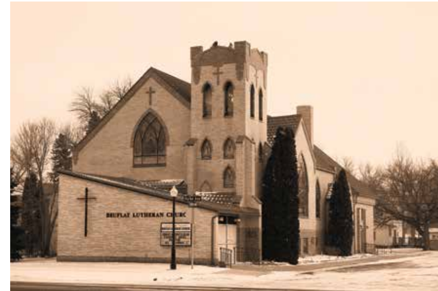
The Bruflat Lutheran Church in Portland received $26,525 to restore its water-damaged church bell tower, whose twice-daily chimes are a mainstay of the community. Courtesy Steve Gunderson
