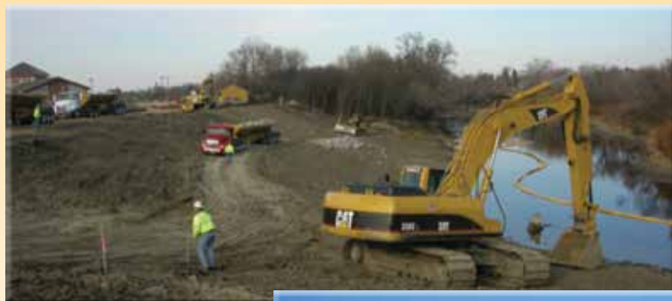
The first loads of rip-rap reach the bank stabilization project at Fort Abercrombie State Historic Site, October 31, 2012. Photo by Paul Picha, SHSND
