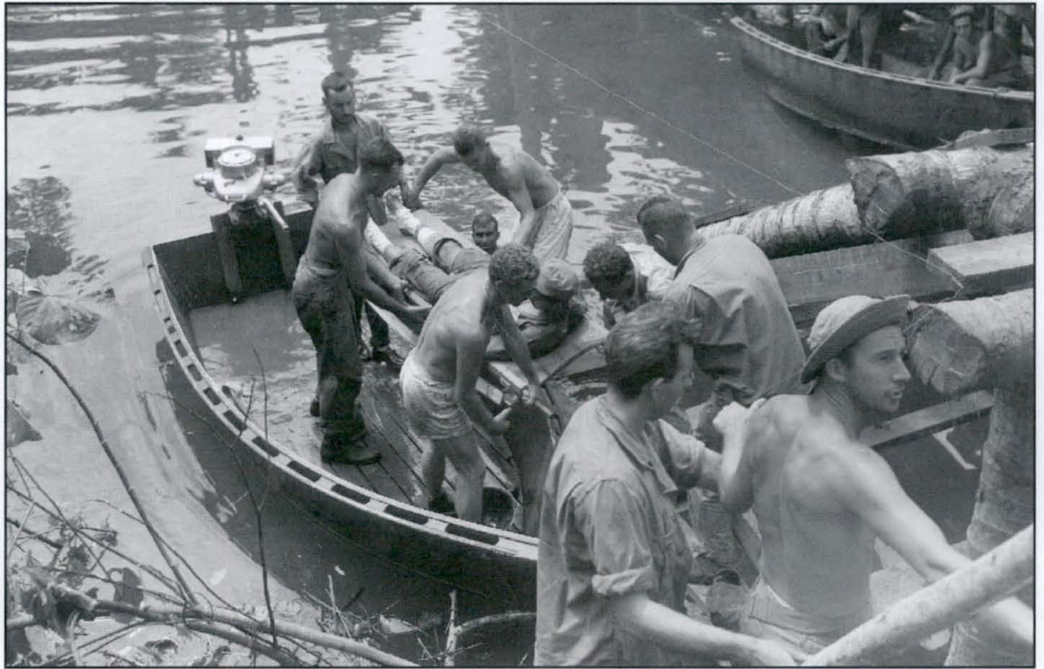
Casualties from front line fighting are being unloaded at scene of new bridge construction on the Matanikau River, Guadalcanal. The first part of the trip was in flat-bottom boats pulled and walked through shallow rapids. The latter half was made by outboard motorboat. U.S. Army Photograph. NDNGHH&A.
