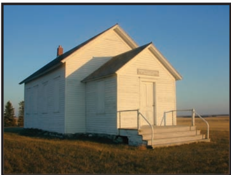
The Ingersoll School was built in Veeder Township near Washburn in 1885 and enlarged in 1903 to serve the growing needs of the community.
