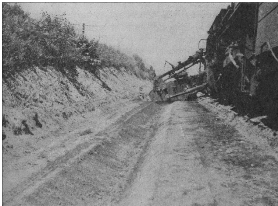
Figure 11. Construction of drainage ditches (Rench 1946:21)
