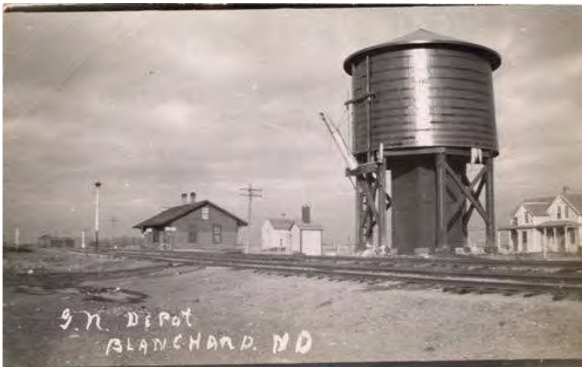
Figure 26. Water tank at Blanchard, ca. 1925 Institute for Regional Studies, North Dakota State University, 2000.56.4
