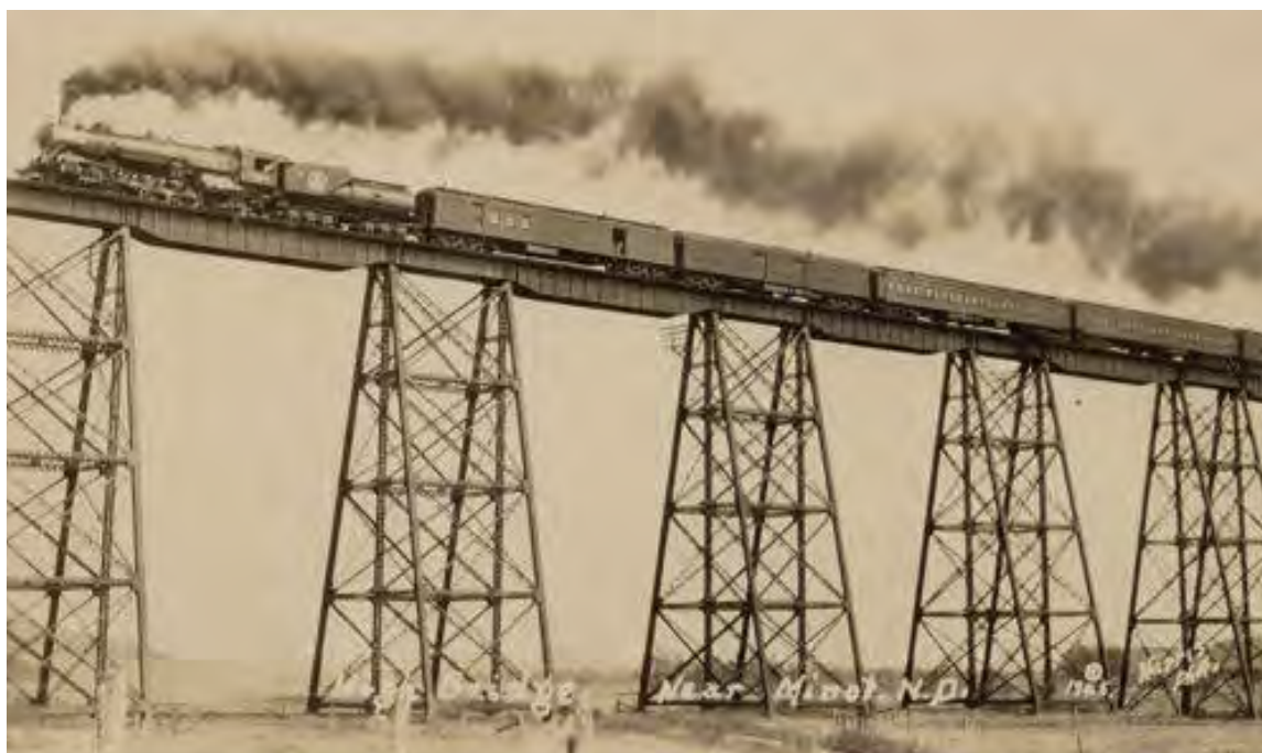
Figure 17. Great Northern viaduct near Minot, 1925 (Institute for Regional Studies, North Dakota State University, 2000.350.108)
