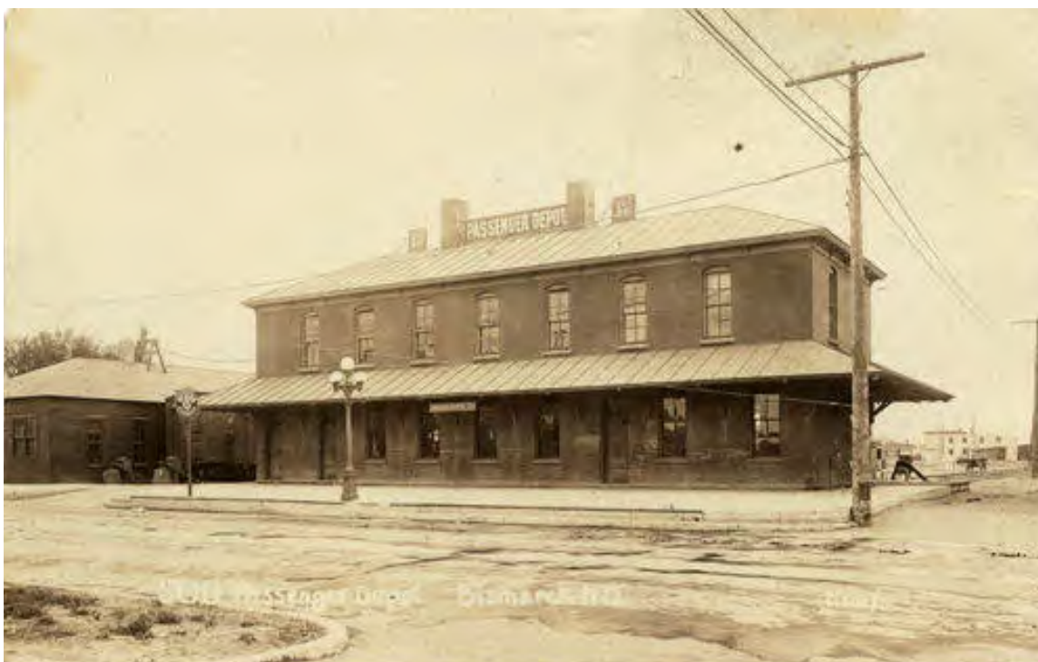
Figure 21. Soo Line large passenger depot, Bismarck, ca. 1910 (Institute for Regional Studies, North Dakota State University, 2000.54.315)
