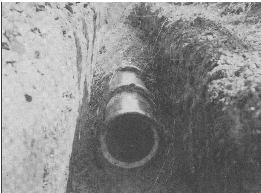
Figure 12. Tile pipe for drainage (Howson 1926:123)
