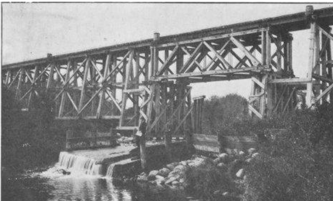
Figure 16. Great Northern trestle at Mayville, ca. 1900 (State Historical Society of North Dakota, A4405)
