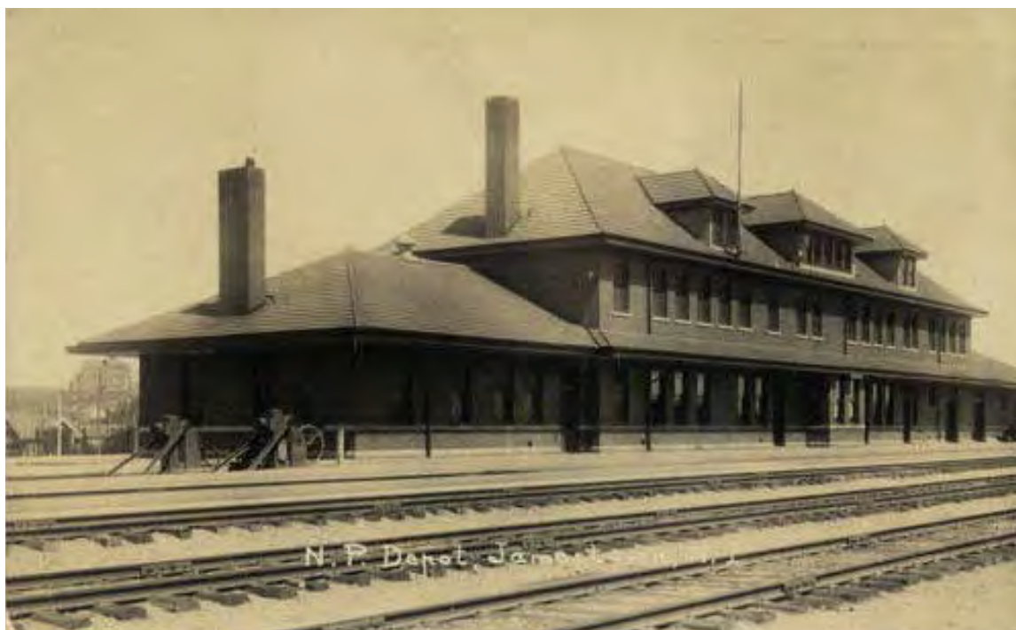
Figure 4. Multiple Tracks at Jamestown Railroad Station, ca. 1910 (Institute for Regional Studies, North Dakota State University, 2000.263.86)
