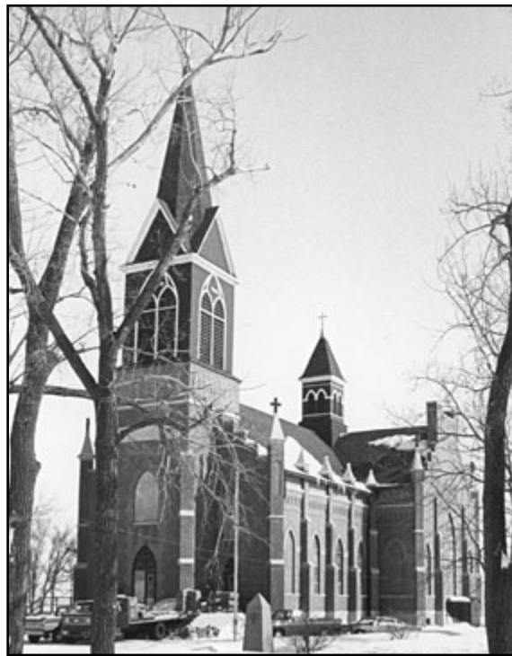
Gothic Revival Style, 32WA2
