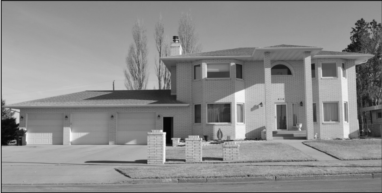
Millennium Mansion, 616 West Avenue F, Bismarck
