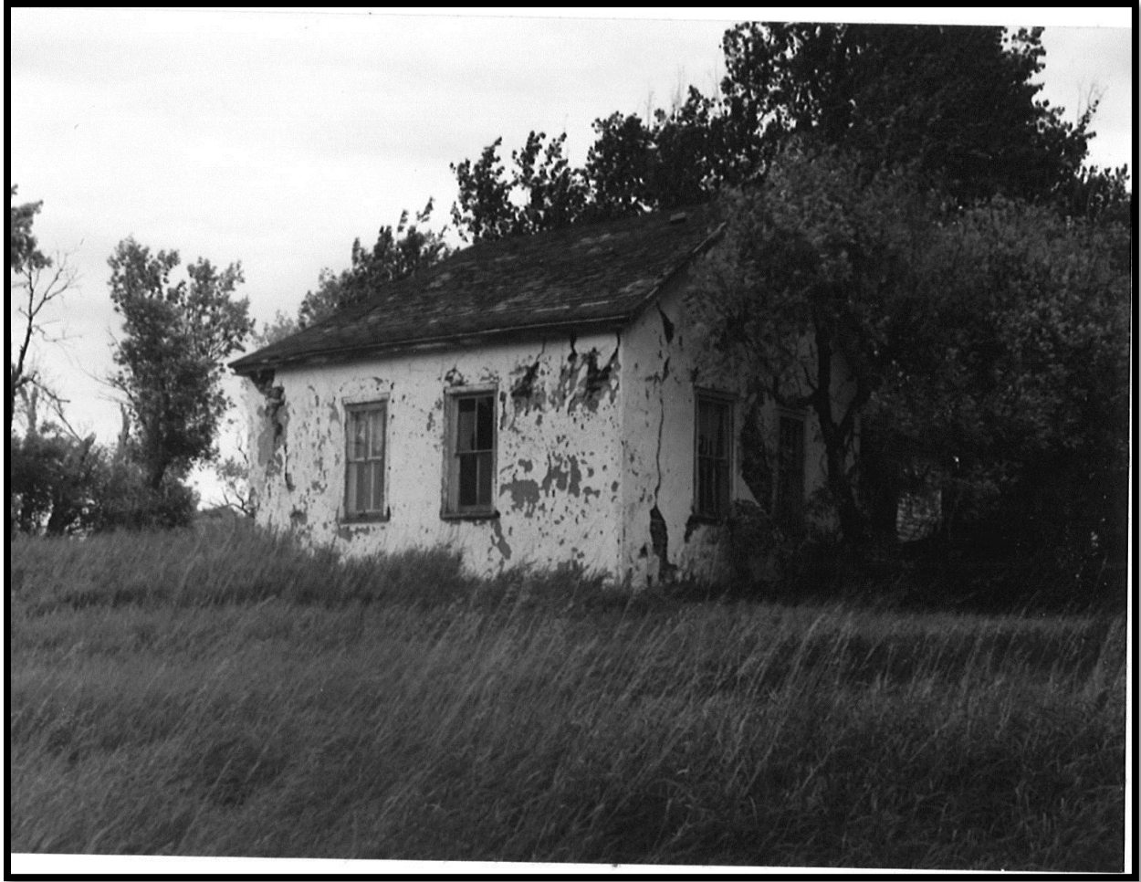
32BA114-Typical example of the house on a German-Russian Farmstead. Materials include earth/clay and uncut stone. Photo Courtesy of Division of Archaeology and Historic Preservation, State Historical Society of North Dakota.
