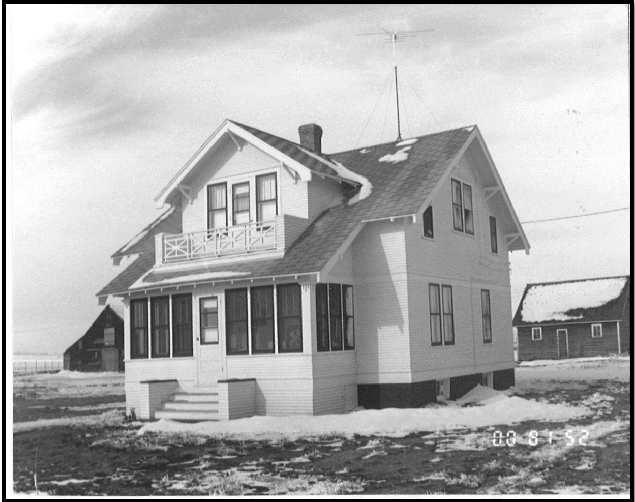
32EM938-This Craftsman style farmhouse in Emmons County, North Dakota was built in 1926. The style is exemplified by the exposed rafter tails and enclosed front porch. Photo Courtesy of Division of Archaeology and Historic Preservation, State Historical Society of North Dakota.
