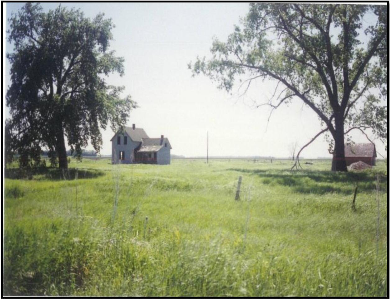
32RI00784-Built in 1882 in rural Richland County, this 2 ½ story square gable front style has a concrete block basement, suggesting that it may have been moved to this site sometime after it was originally built as concrete was not a common material in pre-statehood North Dakota. Photo Courtesy of Division of Archaeology and Historic Preservation, State Historical Society of North Dakota.
