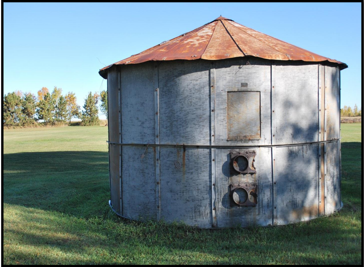
32ML189 Metal grain silo, Freborg Farm, McLean County. Once farmers were able to increase their land holdings due to mechanization, they needed someplace to store excess grain. The use of metal for silo construction was an improvement over the old wood style granaries as it provided superior protection from the elements and vermin such as rats ( rodentia ), house mice ( mus musculus ) and brown rats ( rattus norvegicus ). Photo by Lorna Meidinger, State Historical Society of North Dakota.
